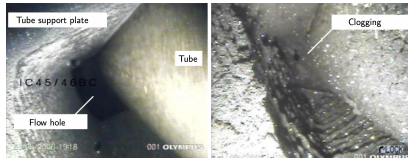
Figure: video examination during an PWR outage (© EDF)
